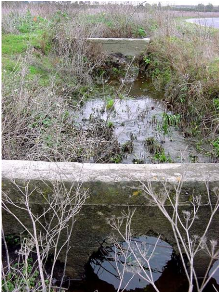
Fig. B.6 Concrete headwalls in drainage
