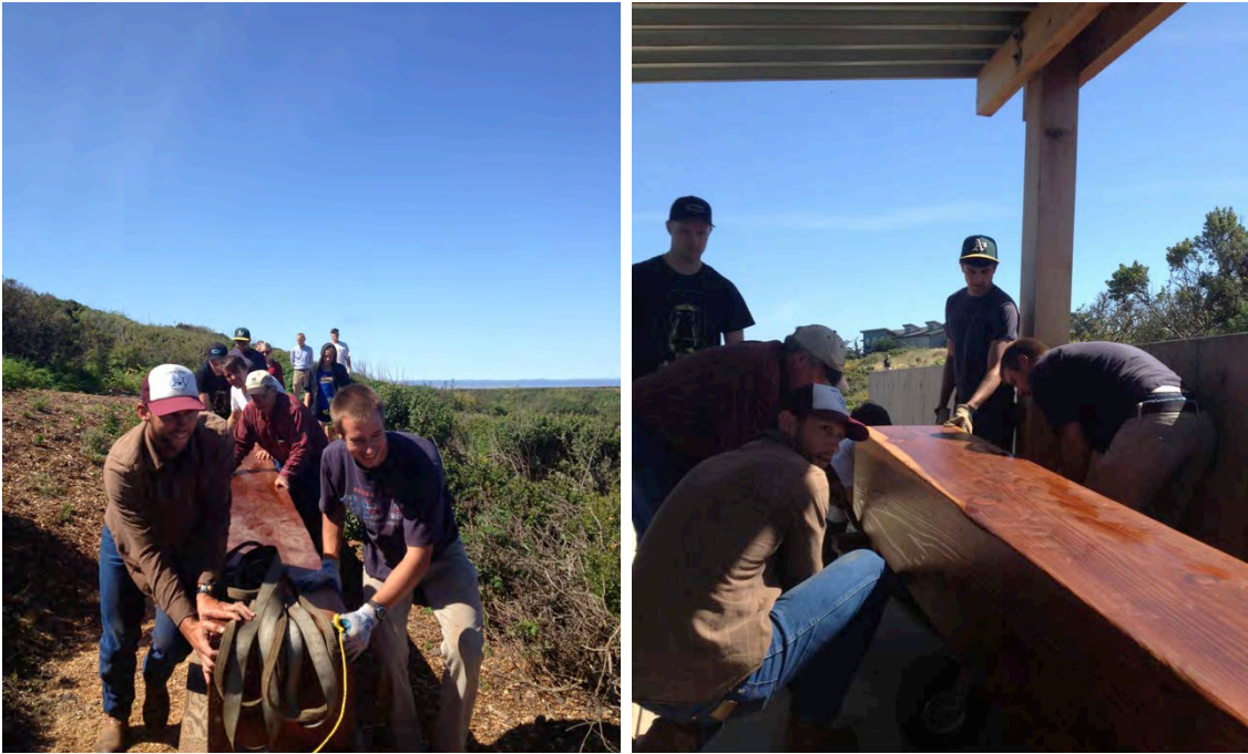
Figure 4. Interns and staff install redwood benches at the Lagoon Overlook Shelter.
