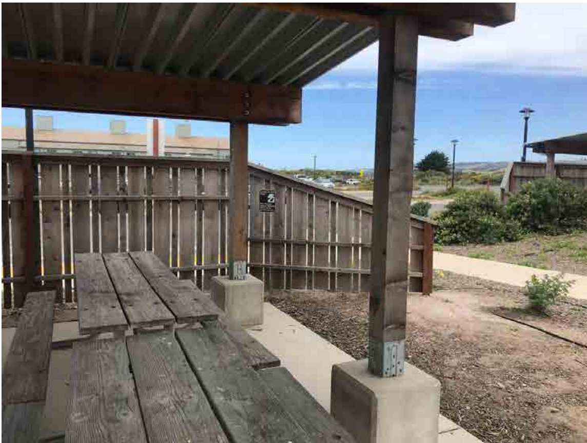
Figure 6. Signage installed at Overlook A.
