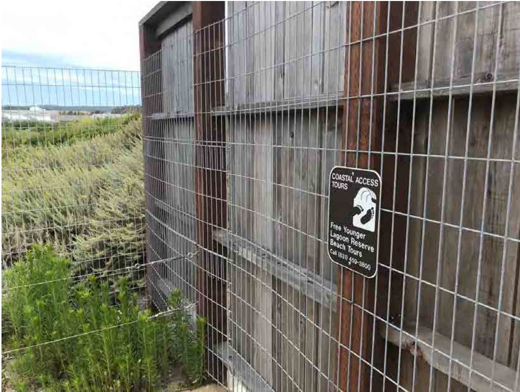
Figure 11. Signage installed at Overlook E.
