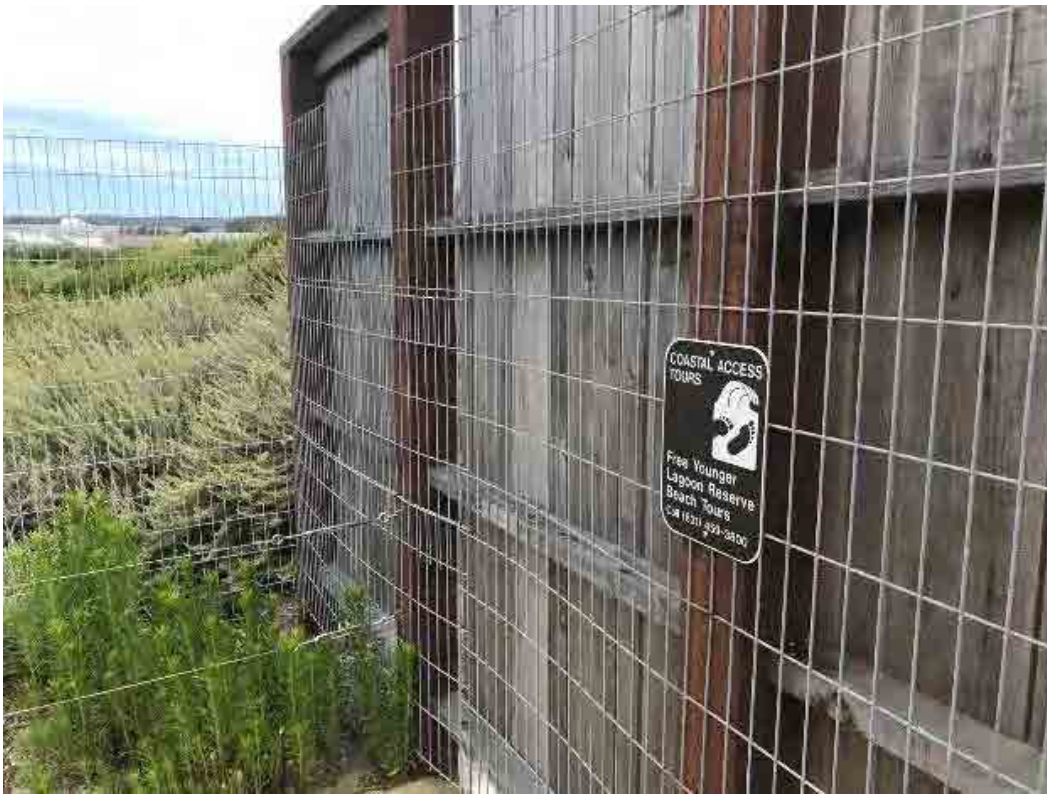
Figure 11. Signage installed at Overlook E.
