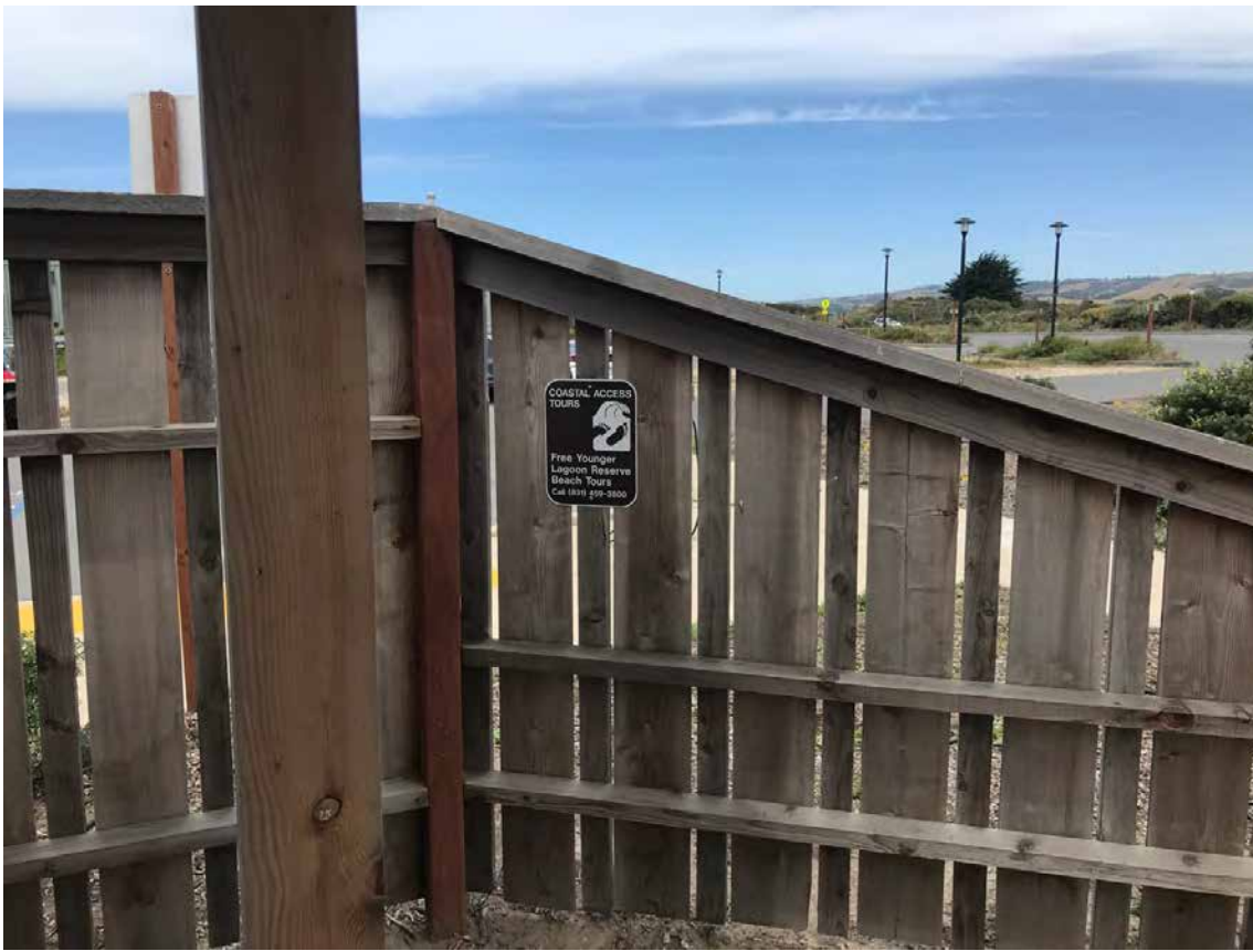
Figure 7. Signage installed at Overlook A (close-up).
