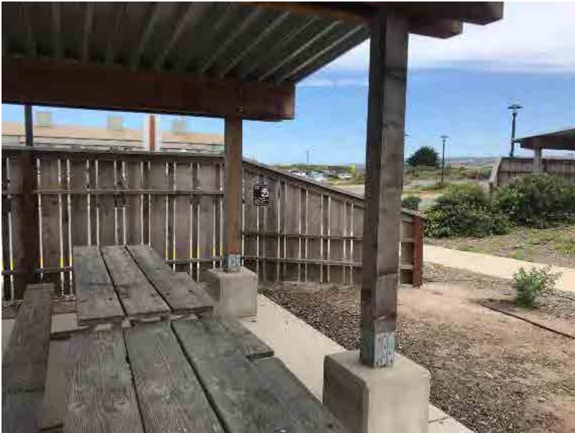
Figure 6. Signage installed at Overlook A.
